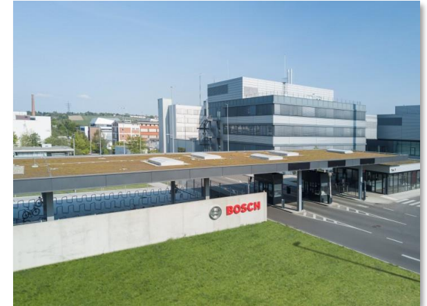
Bosch plant in Stuttgart
